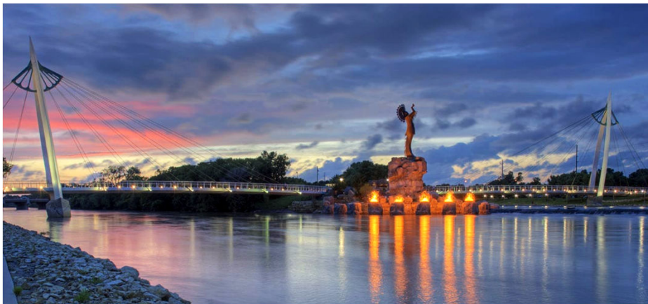
J Keeper of the Plains Pedestrian Bridges / Wichita KS / Blackbear Bosin / Law Kigdon
