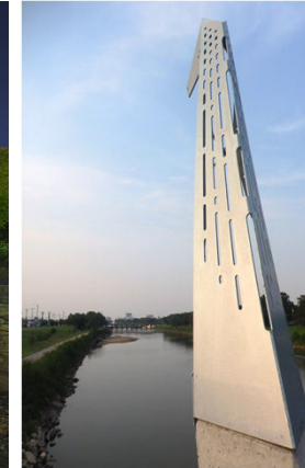
N Blue Heron Bridge / Wichita / WSP / kwED
