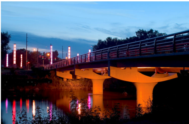
E Sim Park Pedestrian Bridge and Transmission Line / Wichita / PEC / kwED
